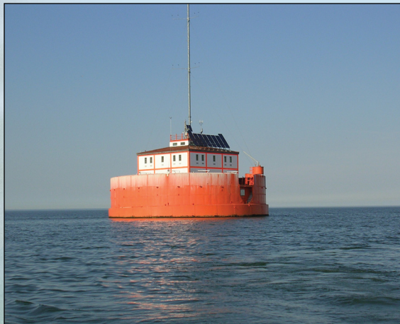
Water intake crib off the coast of Lake Erie in Cleveland, Ohio. LimnoTech's genomic testing will help drinking water plant managers be prepared to adjust their treatment as needed. Photo: Public Domain
